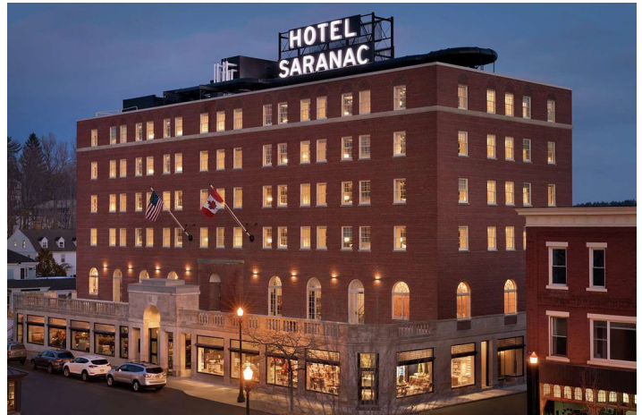
Photo courtesy of Hotel Saranac: The hotel, located in downtown Saranac Lake, adopted a number of energy efficiency and clean energy measures during its restoration process.
